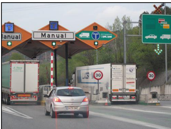
Example of a VIA-T station
