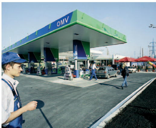
Bulgaria: all our stations are built to international safety and environmental standards.
